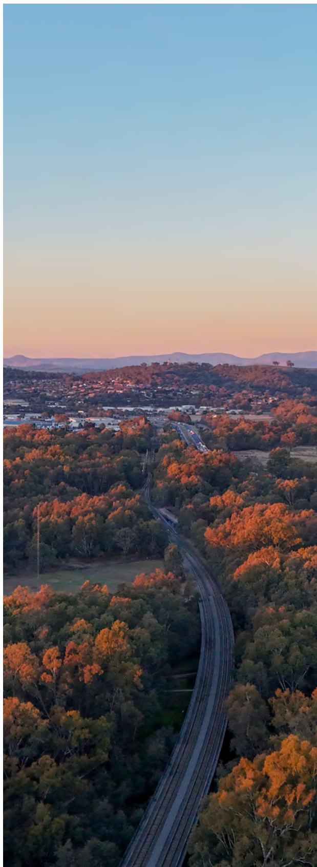
The Country Regional Network links regional NSW to interstate and metropolitan rail systems.
