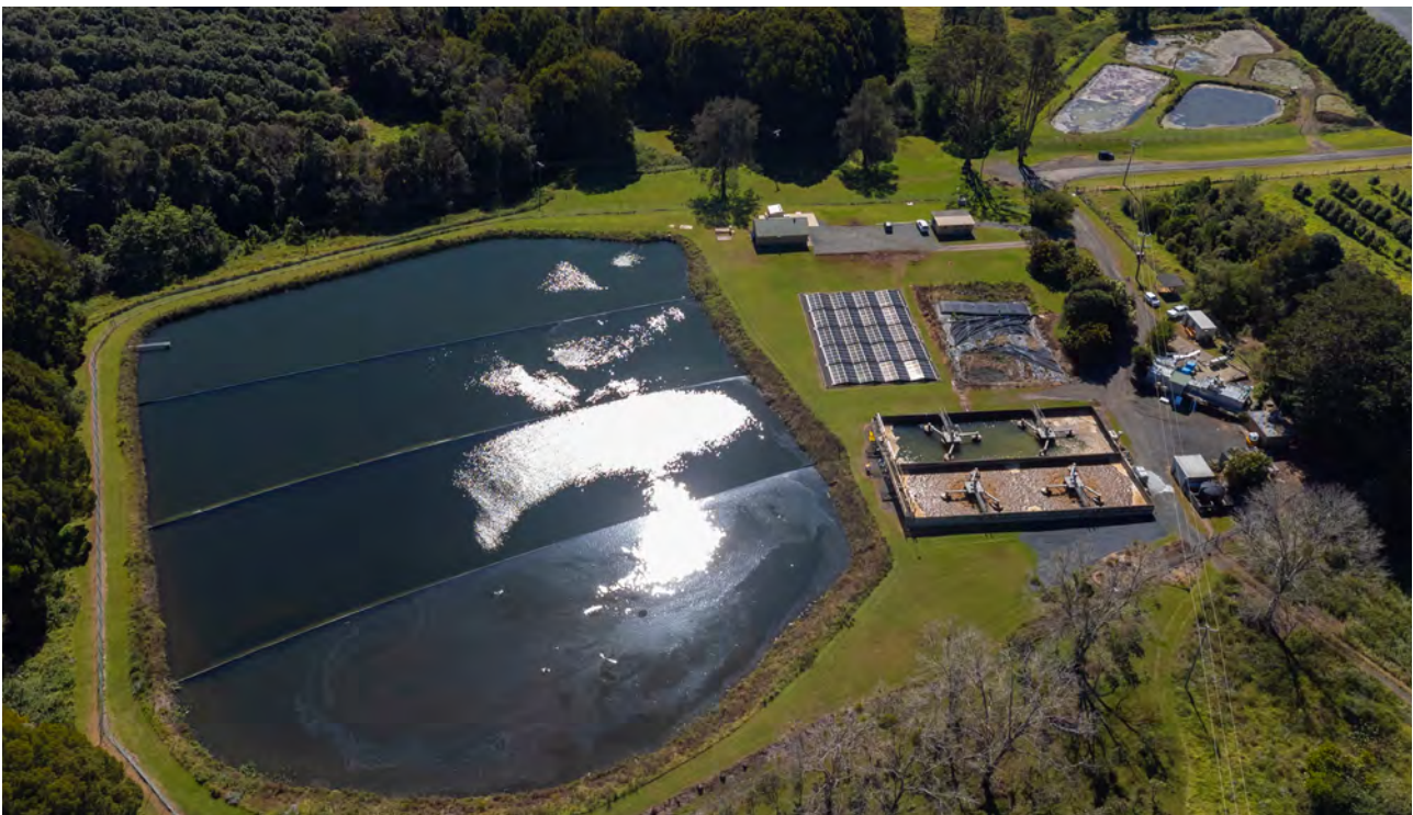
Wastewater can be combined with multiple types of organic waste in a process called co-digestion to boost biomethane production.
